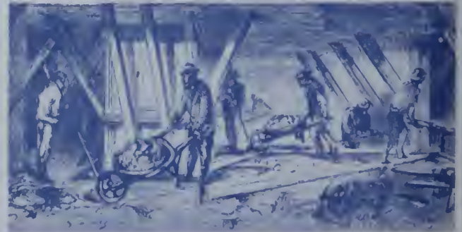
After several fires in the Brooklyn caisson, the Manhattan caisson was lined with steel plate. Excavated material under the caissons was sent up through water shafts.
